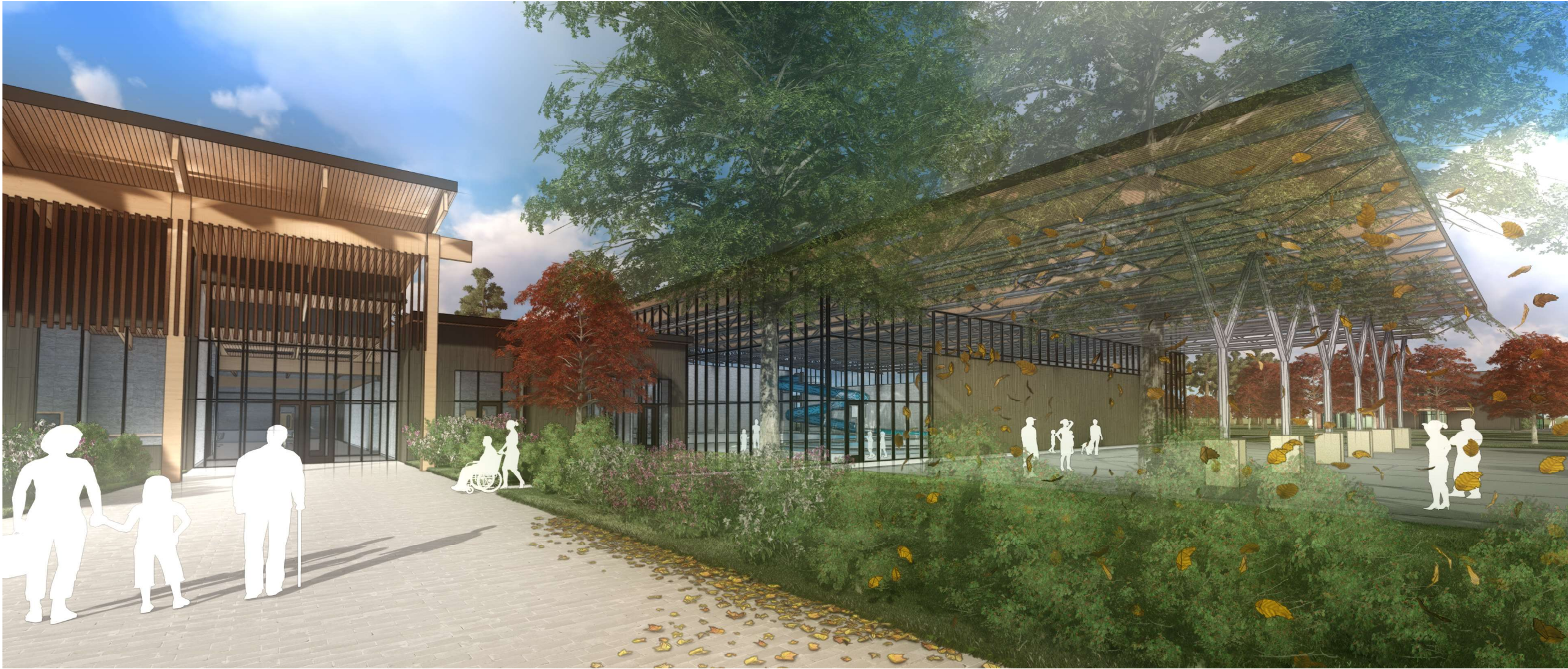
As seen above, the contrast of steel structure and heavy timber is connected with a cross-laminated-timber structural deck. This material adds warmth to the spaces and due to its long-distance spanning capabilities, eliminates many columns. This approach also provides a common aesthetic between wet and dry program areas.
